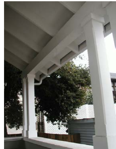
Reclaimed lumber used for porch framing
