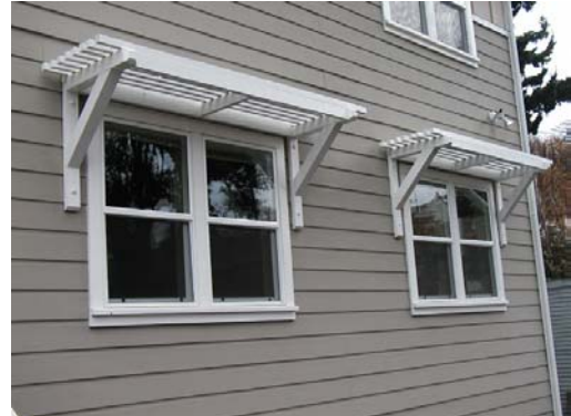
Sun shades on south facing windows reduce the intensity of solar heating
