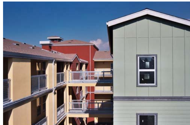
View facing courtyard
