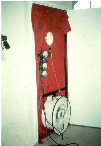
Figure 1. Blower door testing for building envelope leaks
