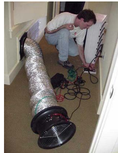
Figure 2. Testing for duct leakage
