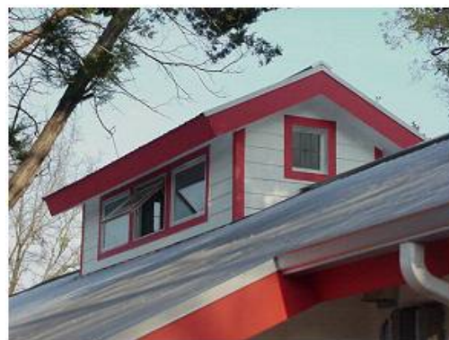
Figure 1. Roof monitor or cupola 1
